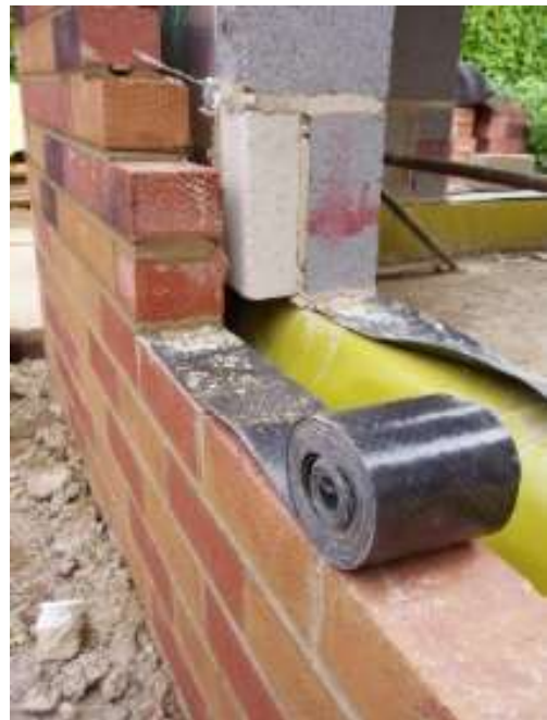
Figure 20: DAMP PROOF MEMBRANE
