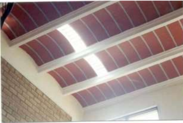
Figure 16: PRE-CAST ARCH PANEL SYSTEM
