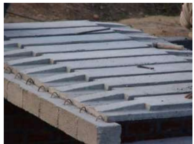
Figure 15: PRE-CAST RCC PLANK AND JOIST
